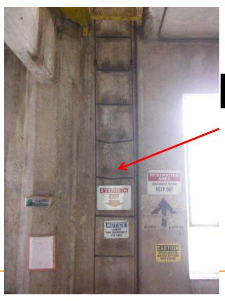
This ladder has bent rungs. Rungs need to be repaired or ladder replaced..
