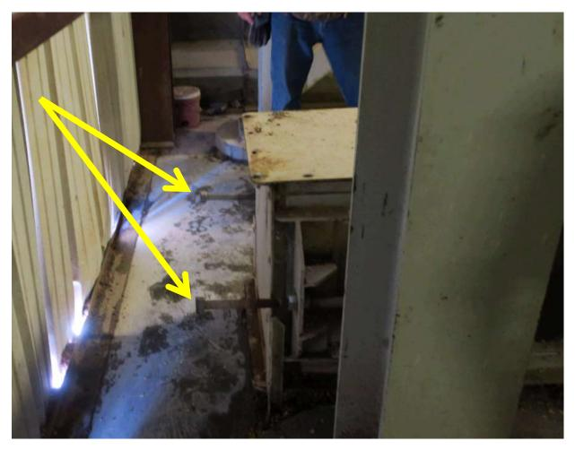
Bolt ends stick out into walkway – trip and laceration hazard
