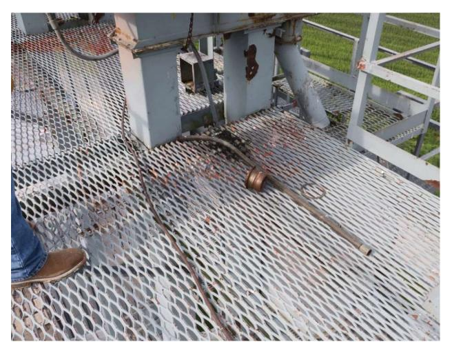
Clutter on elevated walking surface is a severe hazard
