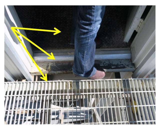
Action: Install threshold to connect the transition between the walking surfaces
