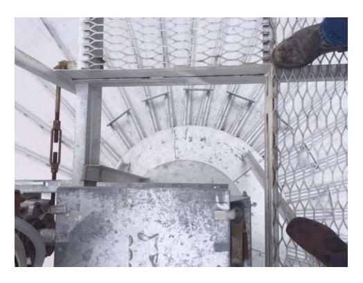
Anyone servicing the motor on this platform needs to step over a floor opening with a fall to the bin top below
